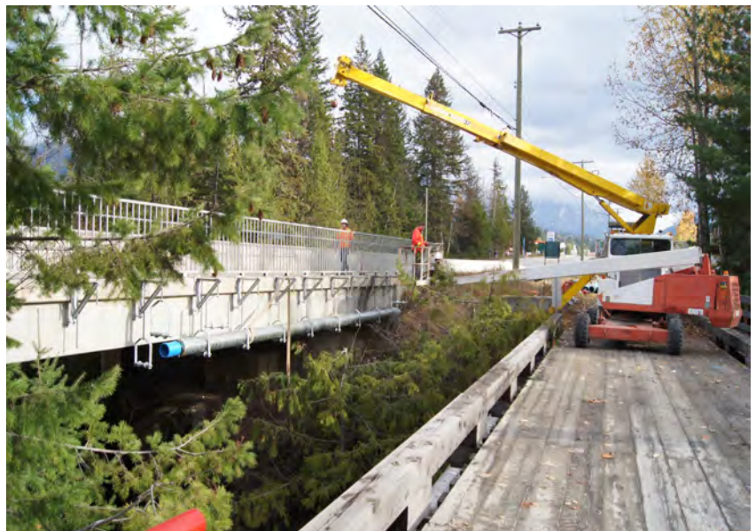
Water line being placed for the Sewer Treatment Plant.
