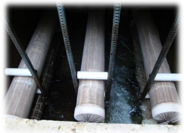
Figure 1 Filter Sock Chamber
