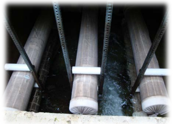
Figure 1 Filter Sock Chamber
