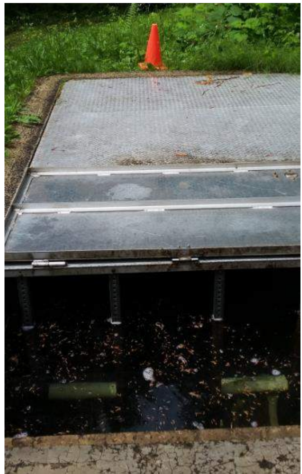
Figure 3 – Upper Brouse Intake Structure (Top: Intake Off Brouse Creek and Covered Filter Sock Chamber, Bottom Left: Intake Off Brouse Creek, Bottom Right: Filter Sock Chamber Partially Uncovered)
