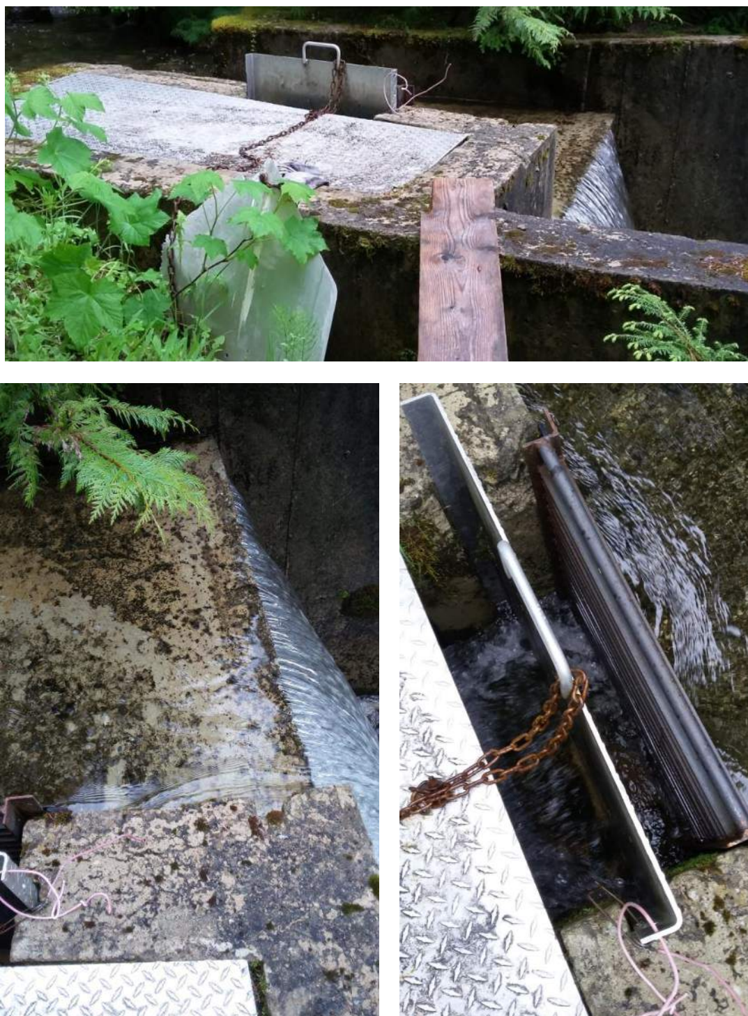
Figure 2 – Halfway Creek Intake Structure (Top: Weir and Intake on Side, Bottom Left: Weir and Intake, Bottom Right: Intake from Above)
