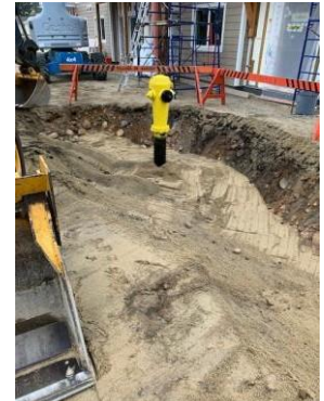
7 th Ave. hydrant installation
