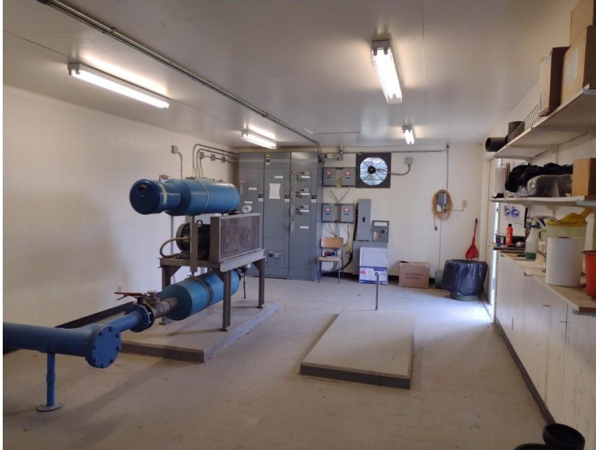
Photo 6 :- View of Mechanical Room (empty blower pedestal not used – see USL Drawing E2)
