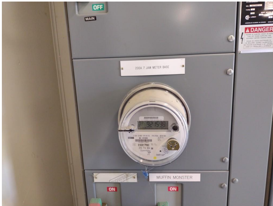
Photo 9: Electrical Meter in Mechanical Room
