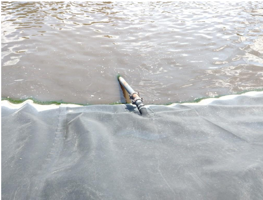
Photo 28: Bend from air feed to lagoon
