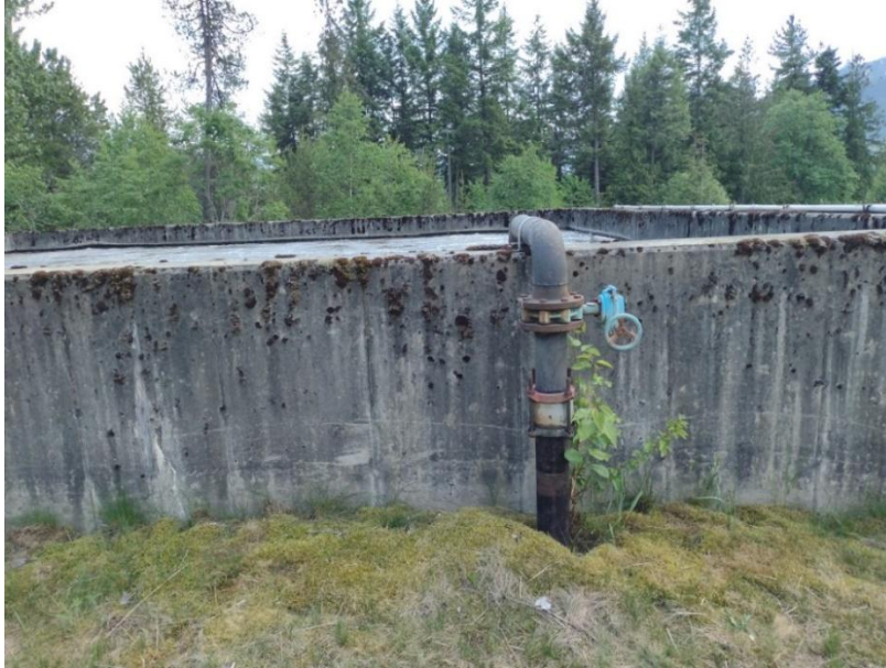
Photo 4: Air valve at CMT
