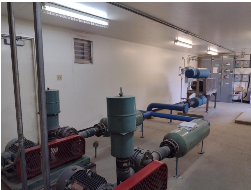
Photo 5: View of blowers in Mechanical Building
