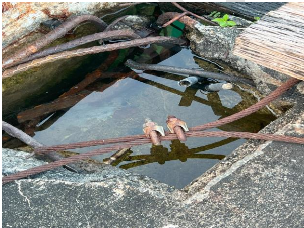
Post tensioning pockets
