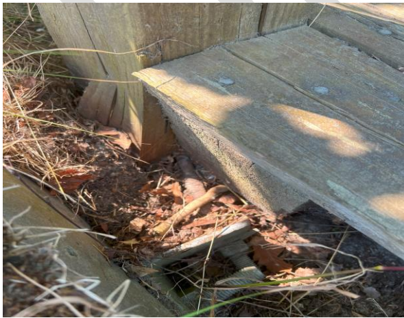
Connection from parking lot to first ramp
