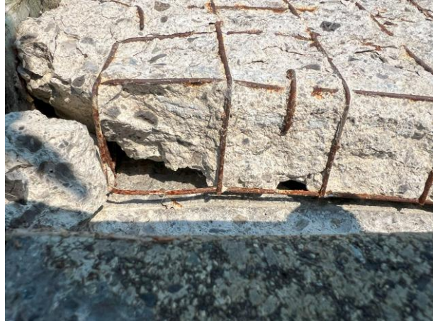
Concrete attachment of pontoons
