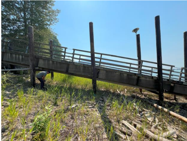
Ramp from parking lot to first marina dock
