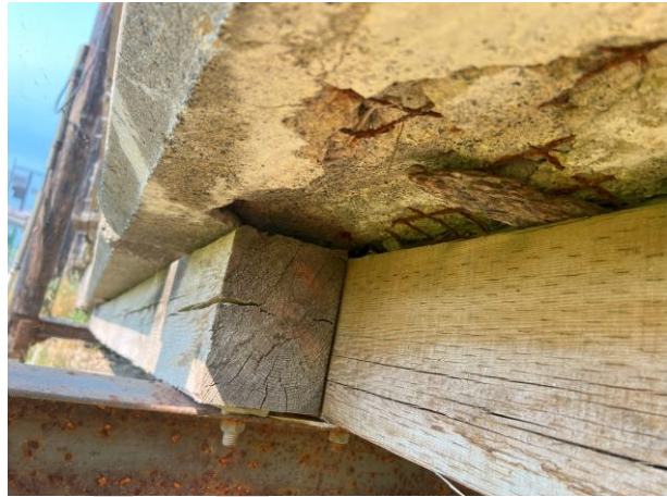
4 th section of access ramp
