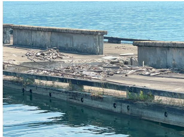
South breakwater mid vertical sections
