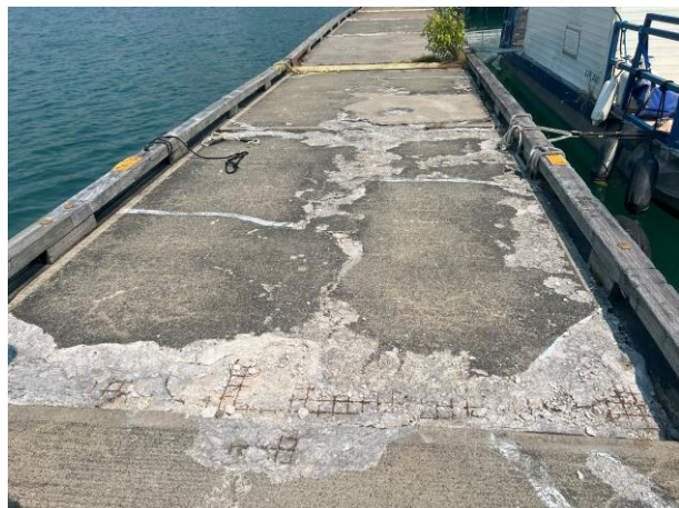
concrete surface on floating docks
