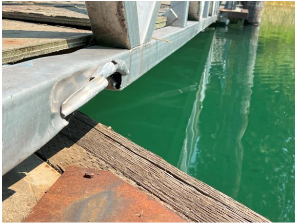
Aluminum ramp from walkway to marina
